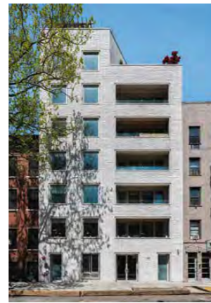
10 355 East 19th Street, Manhattan Architekt: Issac & Stern Architects Fertiggestellt: 2016 Ziegel: K11 Foto: Dean Kaufman
